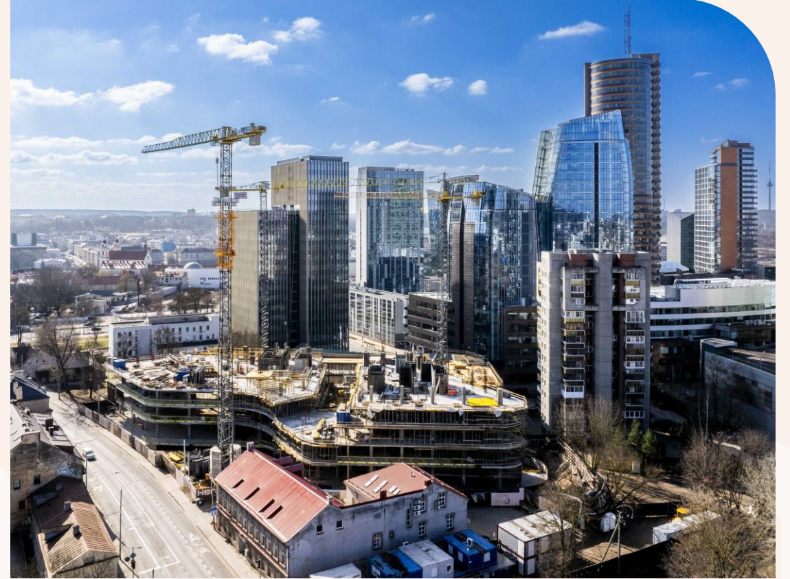
THE 4 TH FLOOR RISES MARCH 2024
