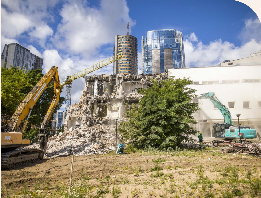
DEMOLITION OF THE OLD BUILDING JULY 2022
