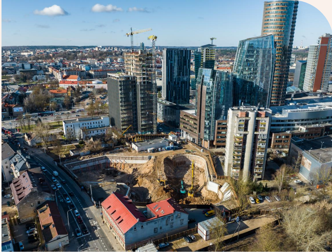
FOUNDATION INSTALLATION WORKS JULY 2023
