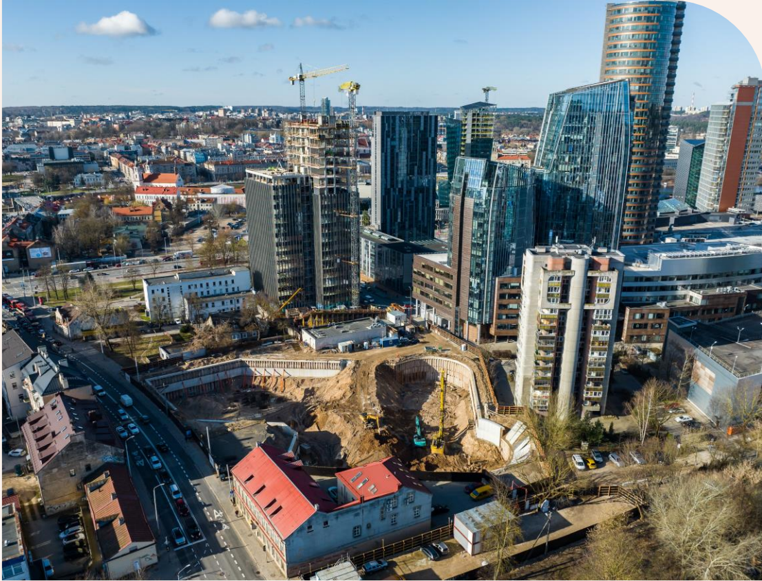
FOUNDATION INSTALLATION WORKS JULY 2023
