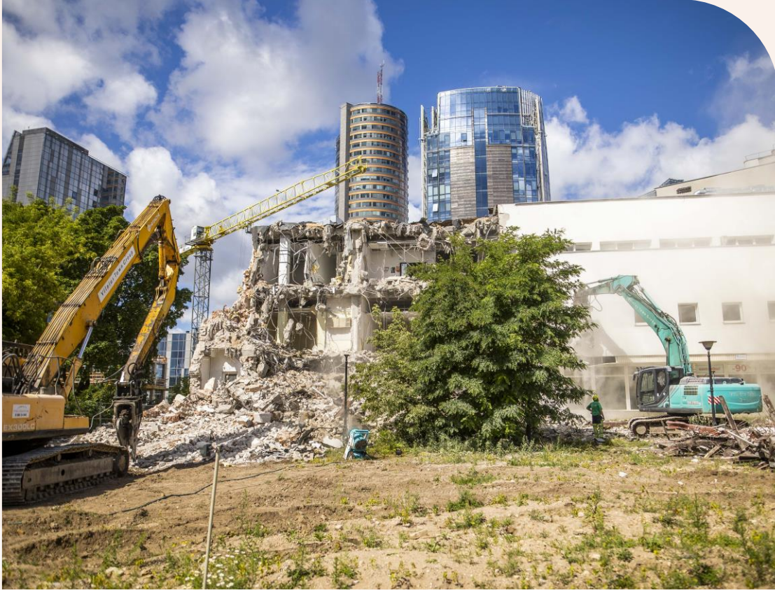
DEMOLITION OF THE OLD BUILDING JULY 2022
