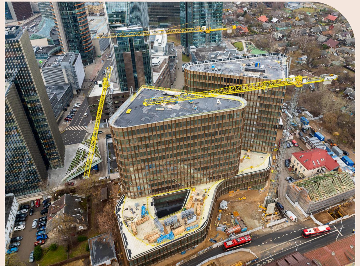
Construction completed, aluminium façade installed – January 2025
